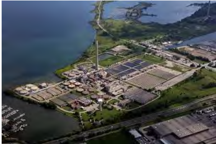
Figure E6-8: Illustration of WWTP site located on shore of Lake Ontario.
