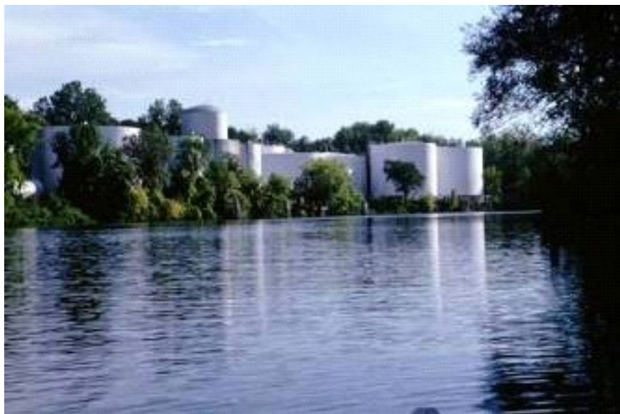
Figure E2.13: Example of Petroleum Fuel Storage near a Water Body
